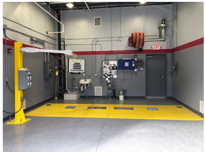
South side interior picture of Chassis Dynamometer building
